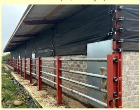
The cattle shed comprises of 4 concrete slatted pens with solid floor lying in area. Externally, there's a covered race and crush with 4 pedestrian doors.
