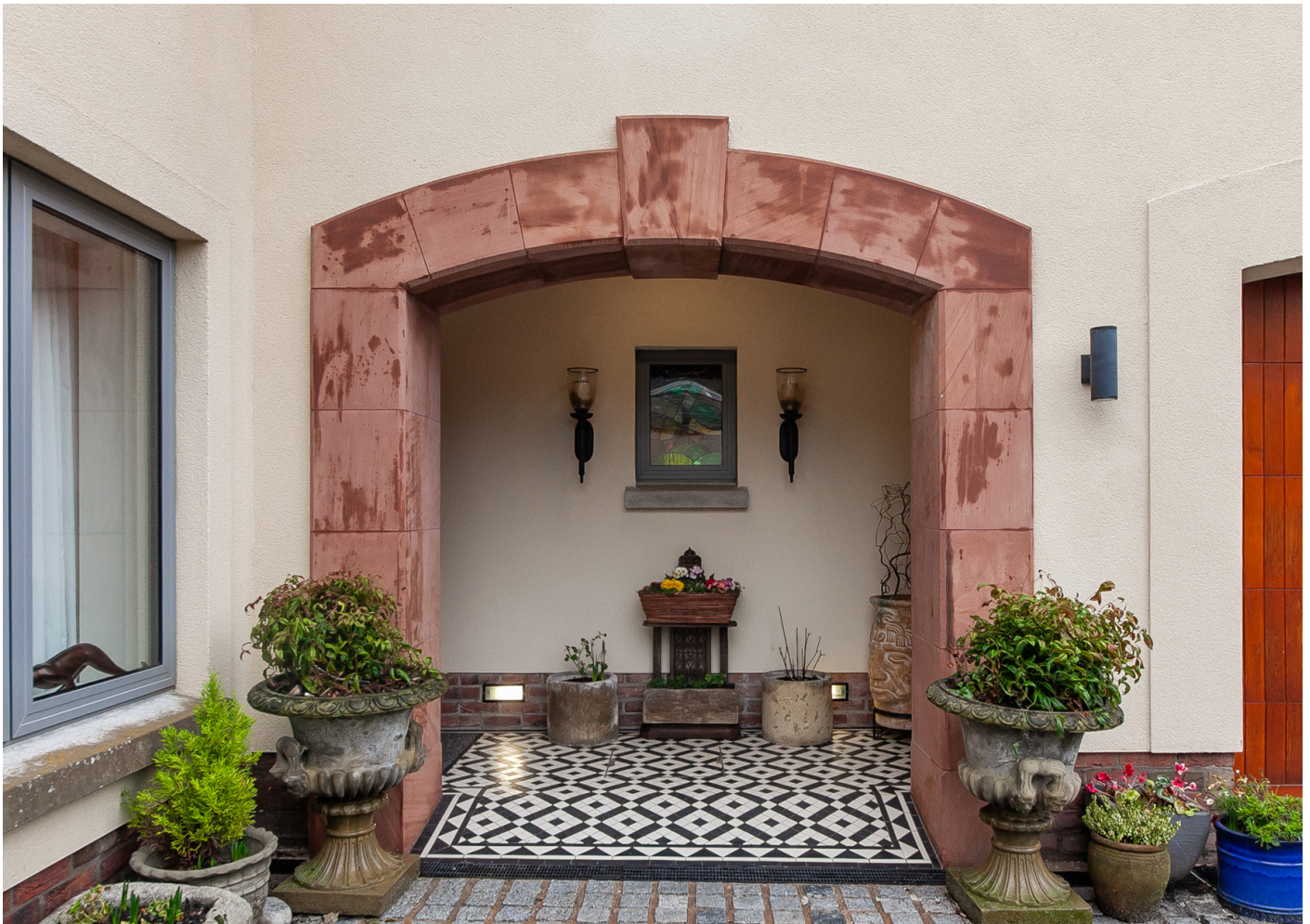
Sandstone detailing to entrance porch EXPERIENCE | EXPERTISE | RESULTS
