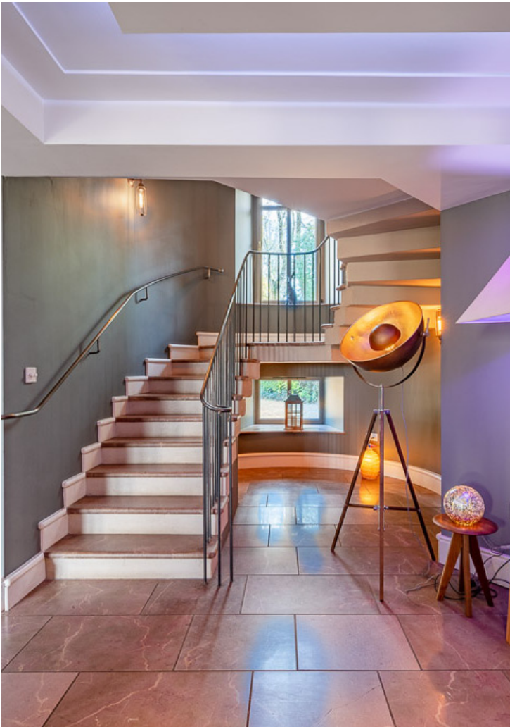
Cantilevered staircase with Armagh marble treads
