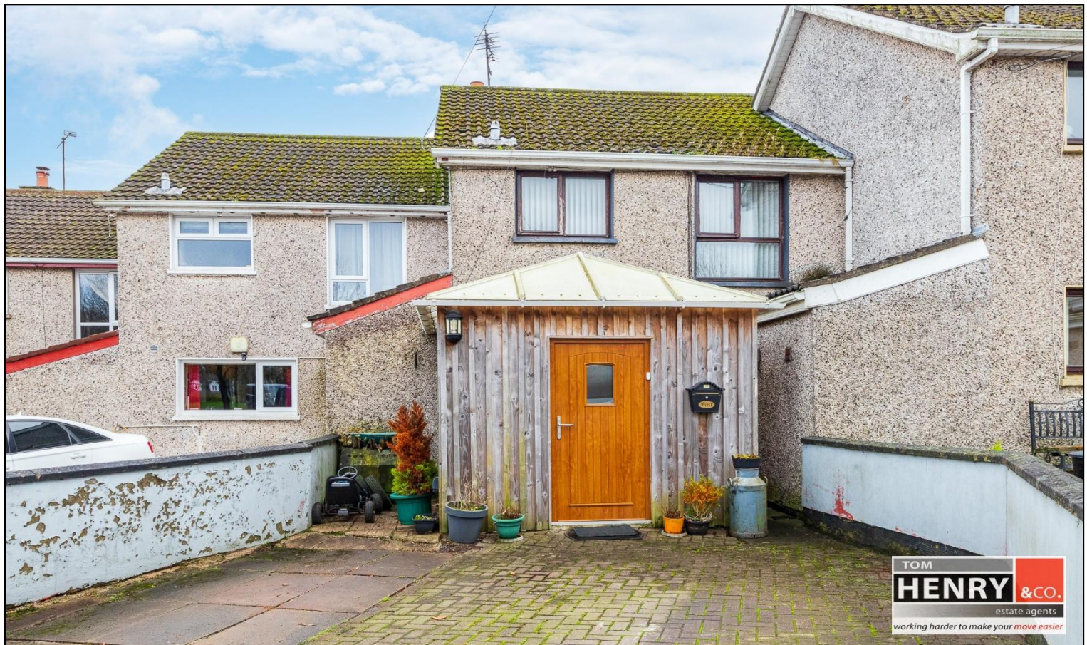
PAVED PARKING TO FRONT. ENCLOSED YARD TO REAR WITH OIL TANK, CENTRAL HEATING BURNER & RANGE OF STORES.
