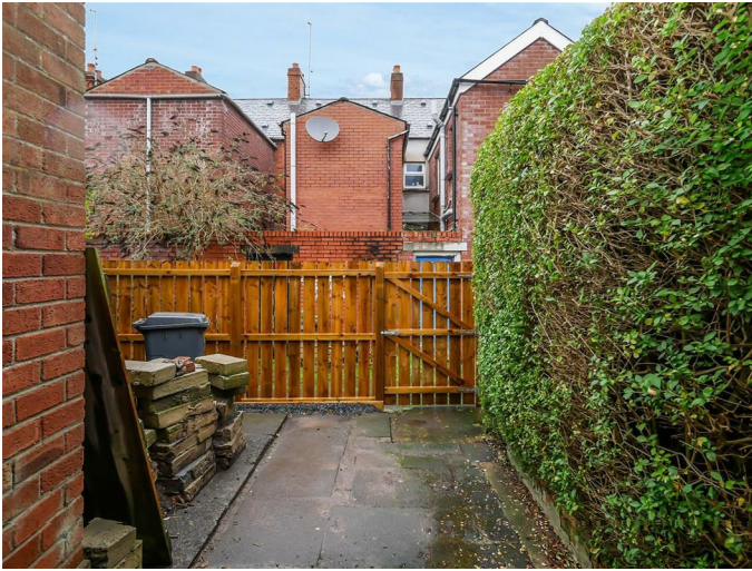
Enclosed rear yard with patio area. Pvc oil tank. Housing oil boiler.
