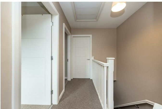
Built-in cupboard with access to gas boiler. Access to loft space via slingsby ladder.
